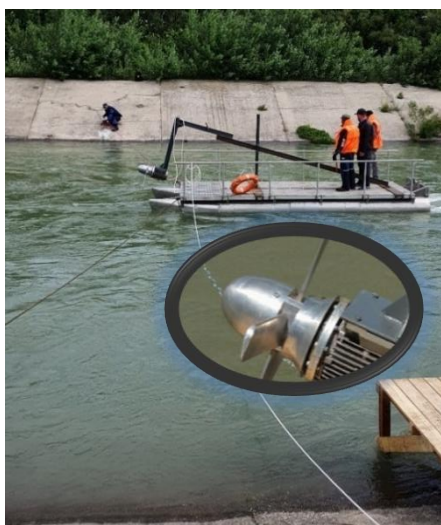
Figure 4. Submerging the turbine in the channel.
