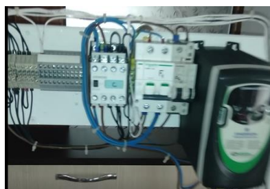
Figure 17. Electrical control and signaling components
